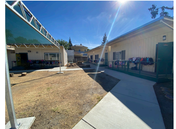
Portable Classrooms at Dingle Elementary
